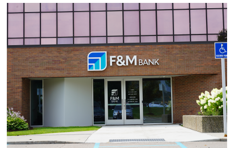
Troy, Michigan Office Exterior
